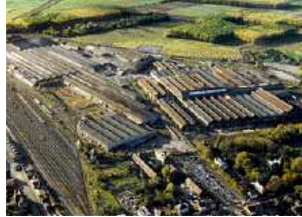
The Crespin facility near the Belgian border : sole plant operated by Bombardier in France
